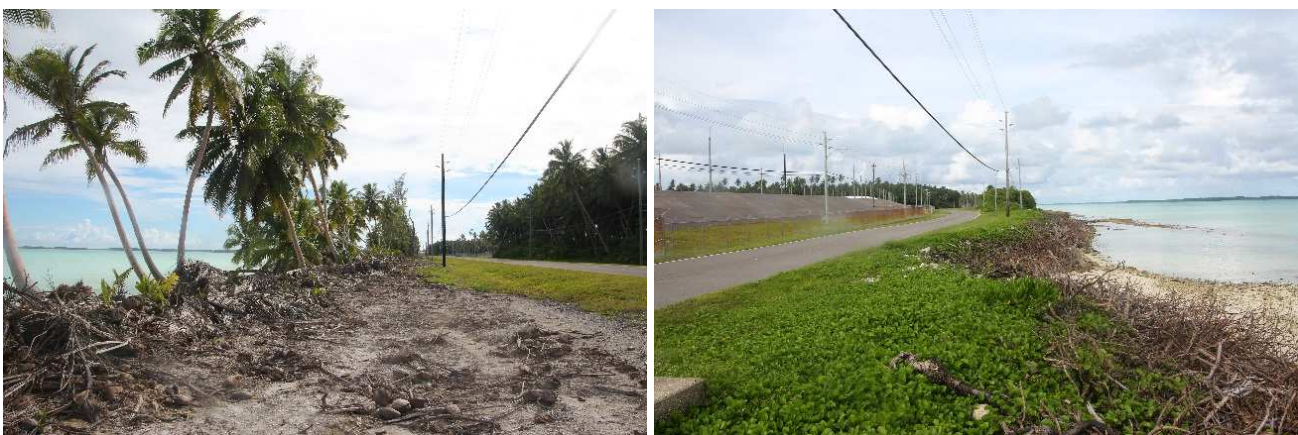
Above: Clearance of coastal vegetation around Mile 11, exposing the road and critical facilities to the risk of erosion and flooding.
