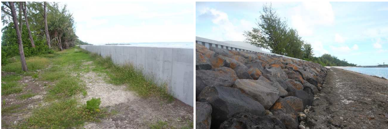
Above: completed revetment work adjacent to the fuel farm, including a new concrete wall (left) above the revetment (right).
