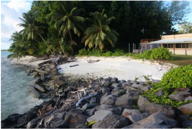
Above: eroding embayment in front of the Reindeer Station, with haphazard concrete blocks to the left which are remains of prior efforts at coastal protection.
